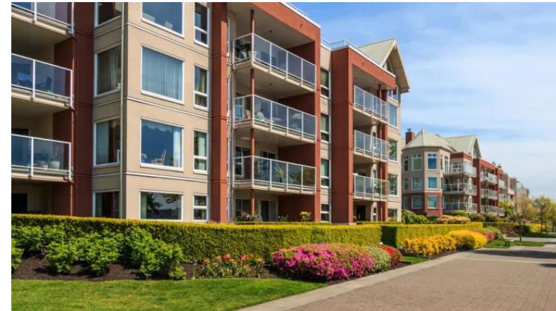
Centralized systems Cascade units
