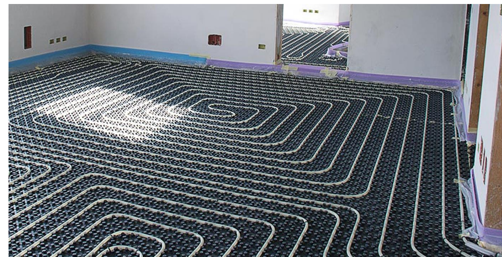
Radiant Cooling / Heating Water at 18°C / 35°C
